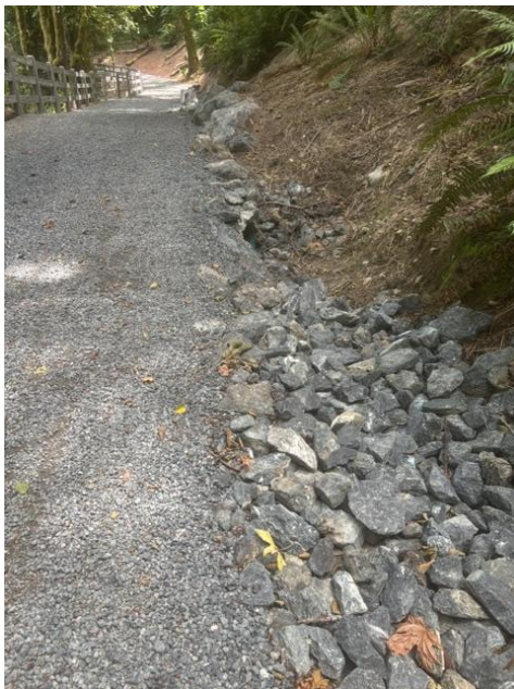
Fig 10: Examples of proper construction of ditches and culverts/pipes
