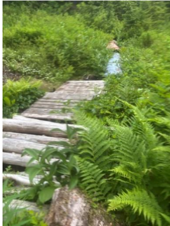
Fig 4: Example of use of shipping pallets (located close to point 3 in map below)
